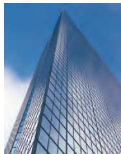
HVAC / Building management
